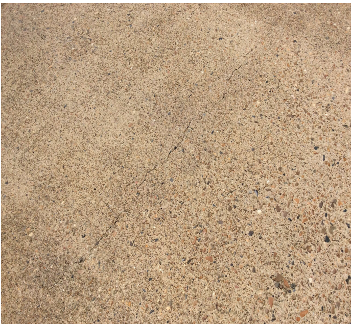
PHOTO 1 Description Unsealed cracks in all spans
